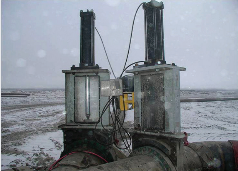
8" Bore ML Series with low temp seals
